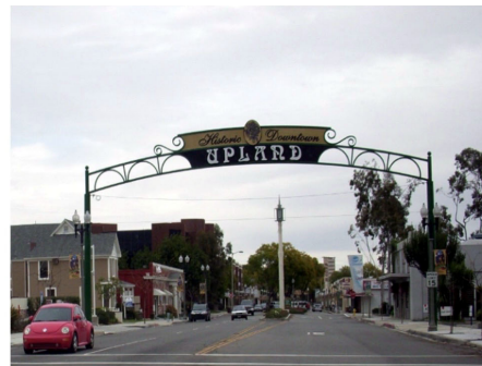
Collector – 9 th St.
