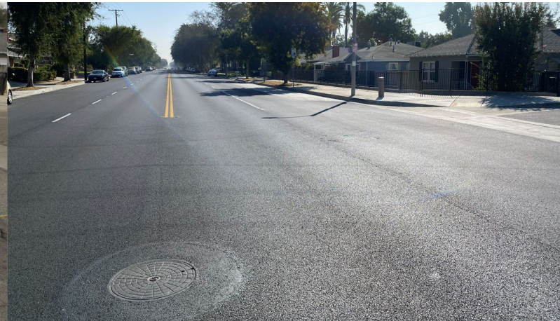
Arrow Hwy at Silverwood Ave: After
