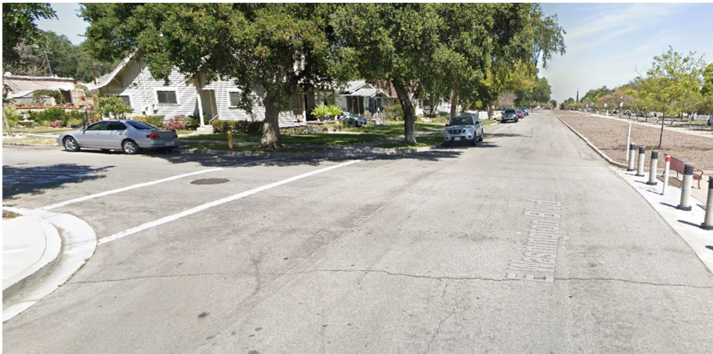
Washington Blvd: Before Slurry
