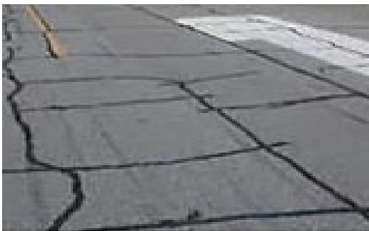
Block Cracking
