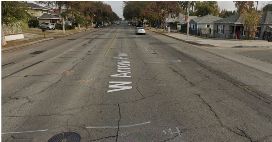
Arrow Hwy at Silverwood Ave: Before
