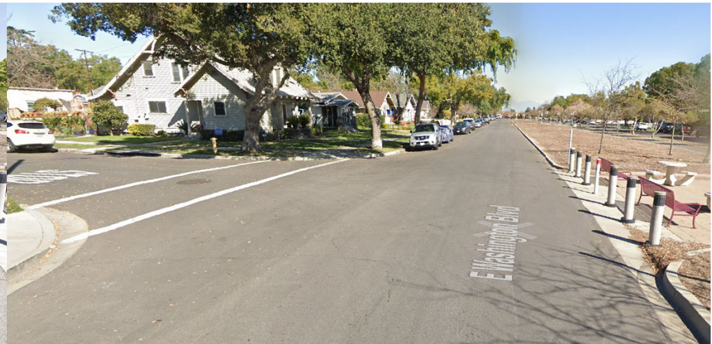
Washington Blvd: After Slurry
