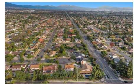
Minor Arterial – 16 th St.
