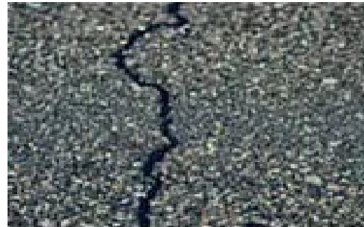
Transverse Cracking
