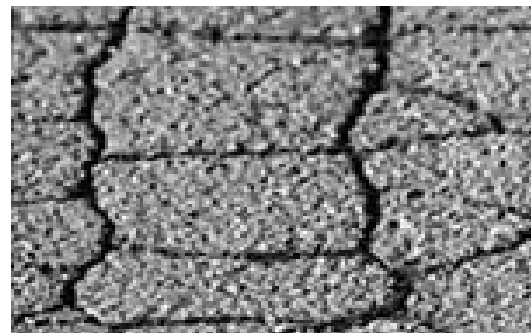
Alligator Cracking
